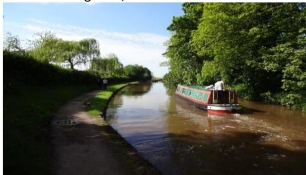
Originally named the Birmingham-Liverpool Junction, and designed to short-cut Brindley's Trent-Mersey Canal; it reduced the journey by 20 miles and 30 locks and goods could then be delivered from Birmingham to Liverpool in 45 hours. Telford changed from the methods of earlier canal builders and, instead of following the land contours, cut his canal on a direct line. This resulted in deep cuttings and steep embankments which can be seen along the tow path.
